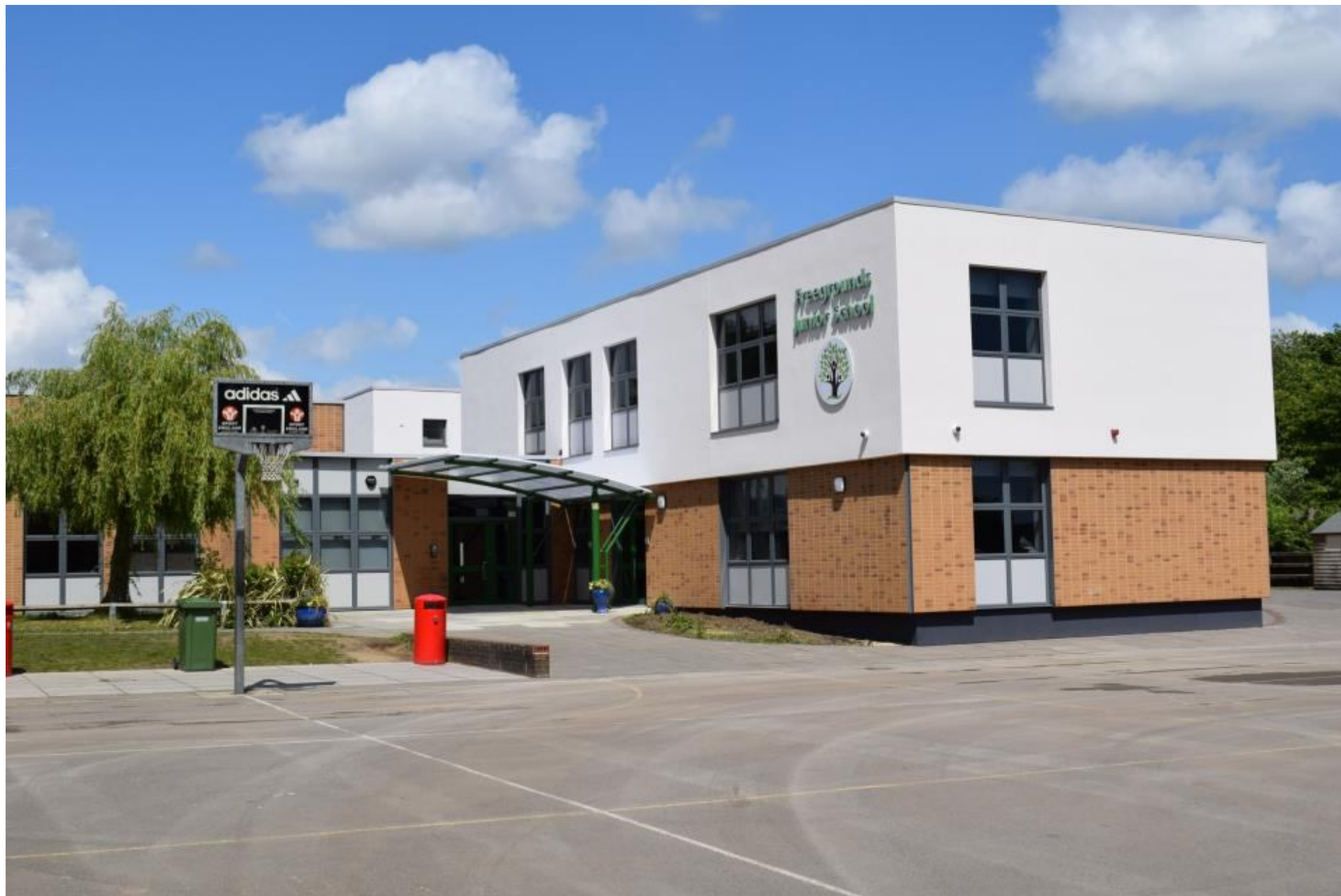
Scola Re-cladding Freegrounds Junior School
